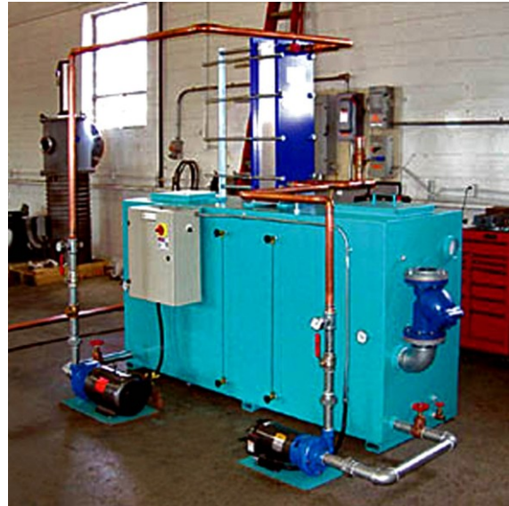
Furnace-coolant reservoir installation
