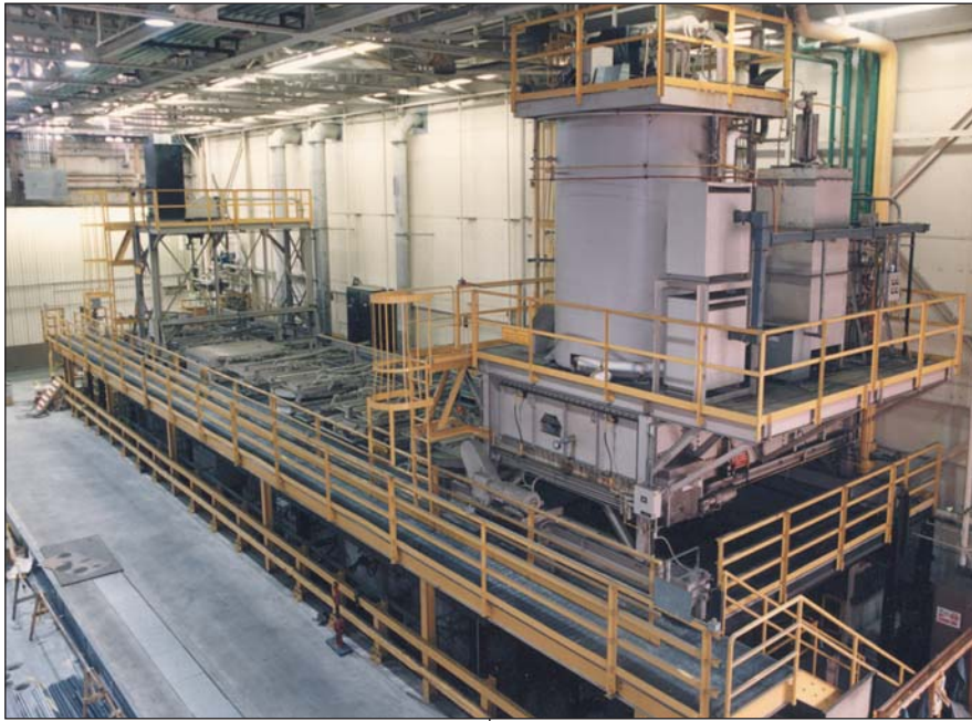
Figure 1 – Large gantry-type furnace used for heat treating landing gear.
